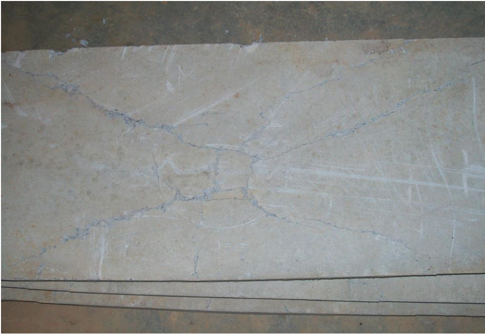
Plate 8: Crack pattern for Solid Slab S2 supported on all 4 sides
